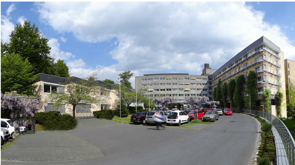
fire safety retrofitting 'Aggertalklinik' hospital, Engelskirchen
