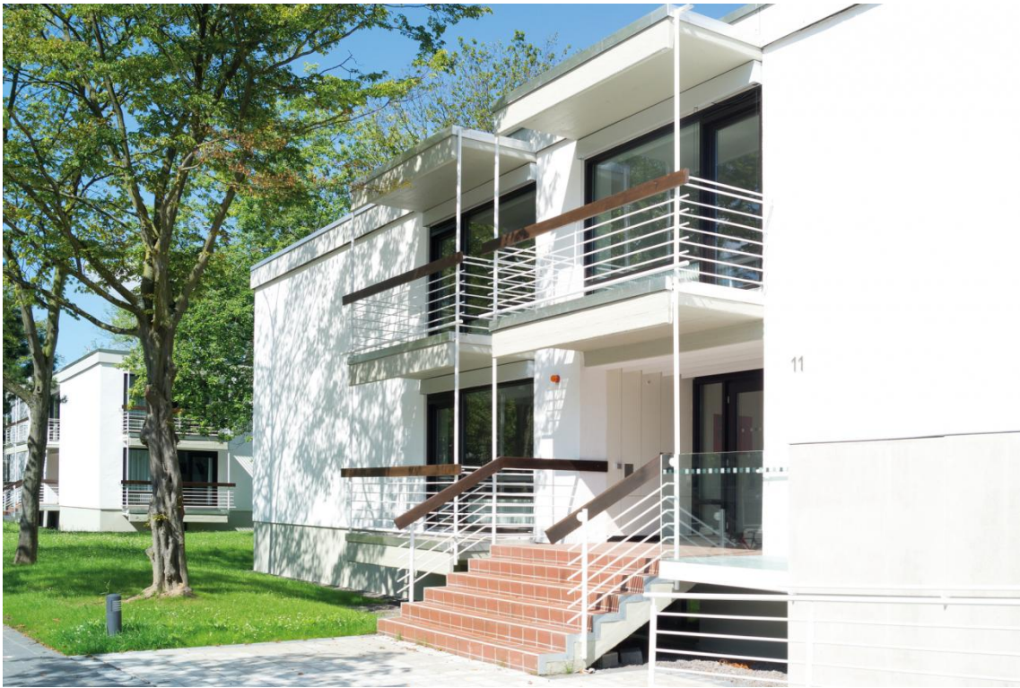
exterior view, office building ('Haus 11')
