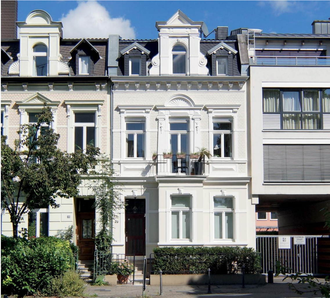
conversion and modernisation, apartment building, Bonn
